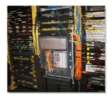
Coastal Technical Services (CTS) recently completed consulting and restoration services for a large Federal Government datacenter. After the datacenter became operational with a large quantity of networking and storage units in place, the datacenter employees noticed a residue accumulating on the equipment surfaces. The residue was traced back to the building environmental control systems.
